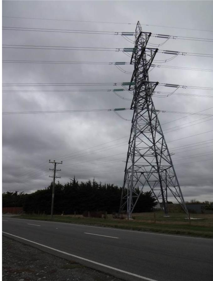
Photo 1 – Comparison of 220kV versus 33kV structures
